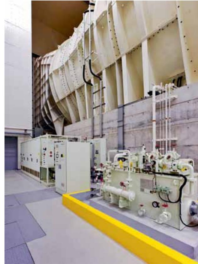
01 The exterior shell of the wind tunnel
